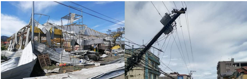
Photo: Damages in infrastructure and disfigured power lines in the streets of Surigao City. (Credit: Emelou Dumas)
