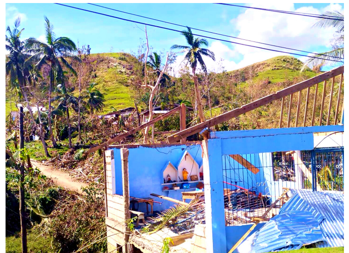
Photo: Totally damaged houses in one of the hardly hit barangays of 2nd district in Bohol. (Credit: Retchel Sasing)
