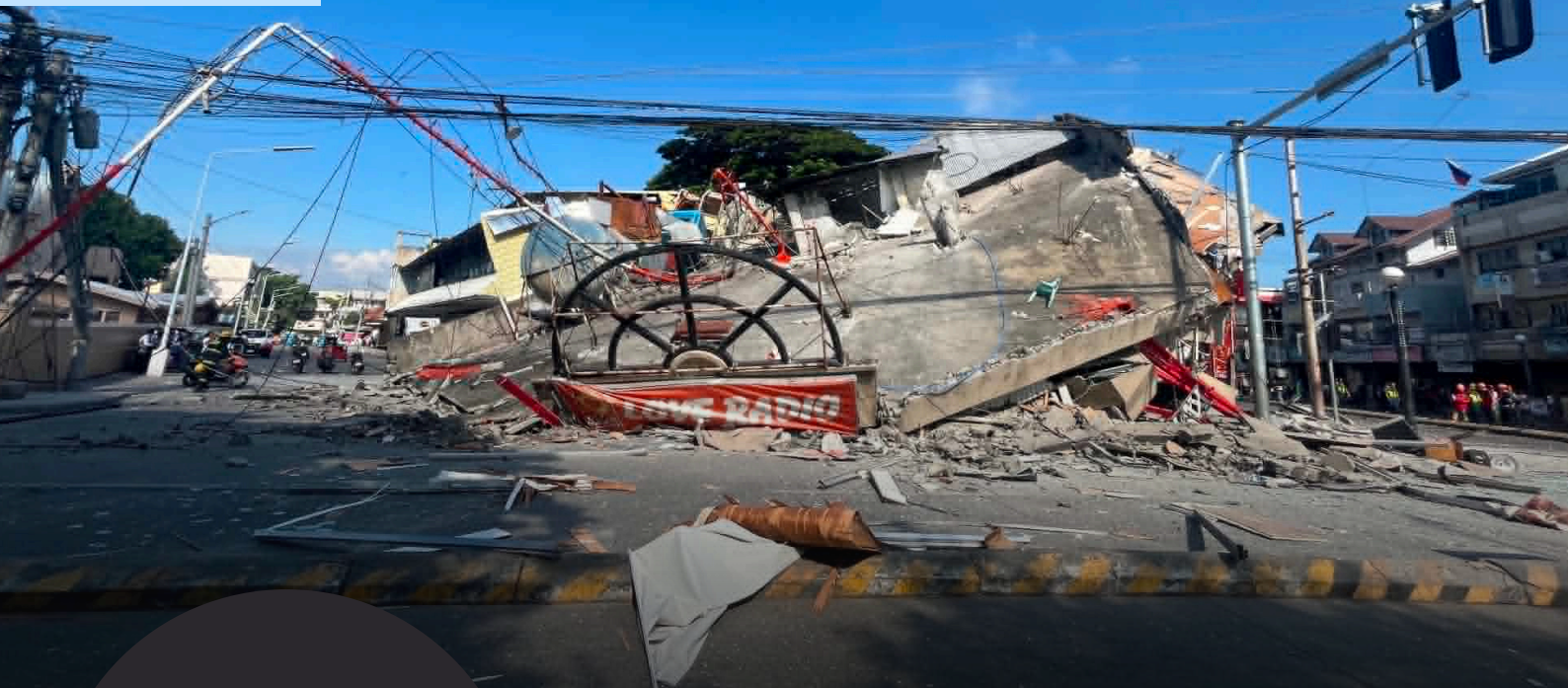
A look at the flattened structure that housed 101.5 Love Radio General Santos, which completely collapsed during the powerful magnitude 7.8 earthquake that struck Mindanao on Monday morning, June 8, 2026 | Photo courtesy of Inquirer
